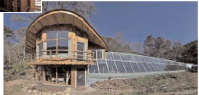
Roald Gundersen built his home and greenhouse (above) using whole trees for structure and support.
